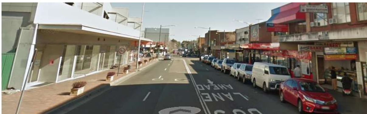
Figure 10 - Scott Street (Westbound towards Macquarie Street)
